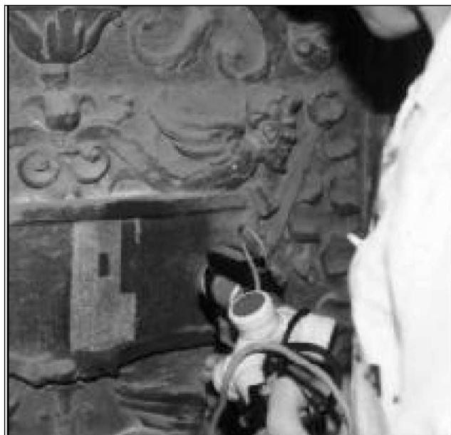
Fig. 2 Q-switched Nd:YAG laser device, operated on porous limestone (calcarenite) during cleaning at Granada Cathedral (Spain).
